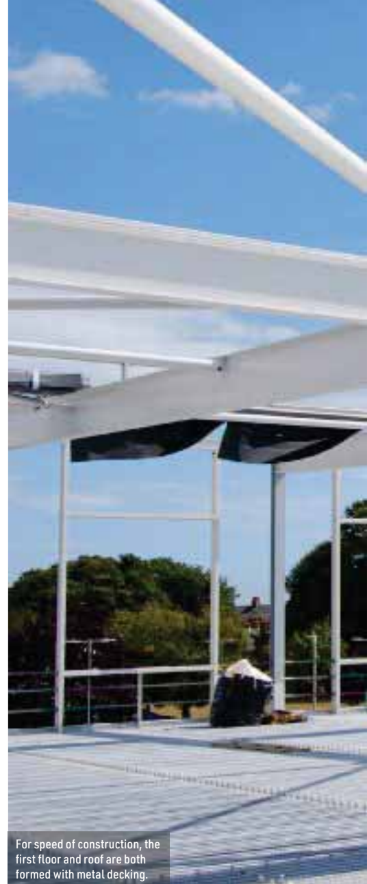
The new facility is accommodated within a two-storey steel frame.
