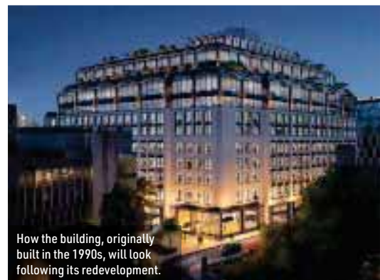
In many areas, new steel columns are connected to existing steelwork.
