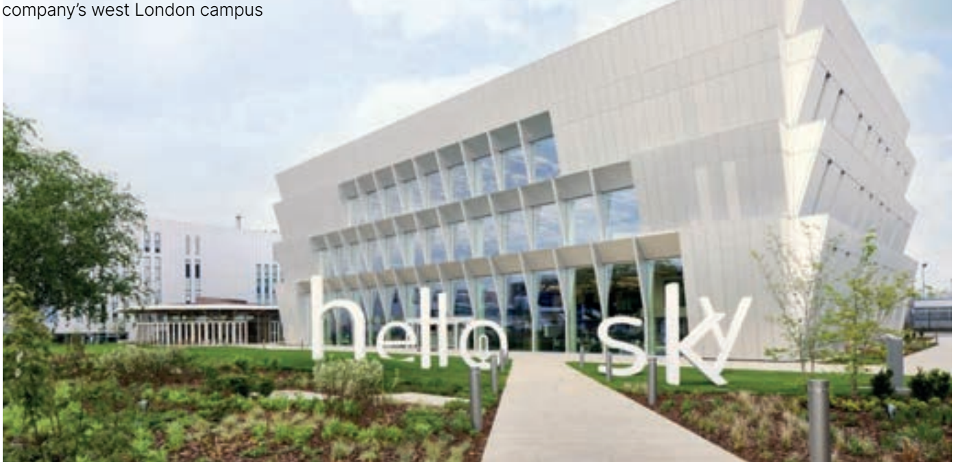
▲ The ziggurat-style facade makes use of splayed columns
