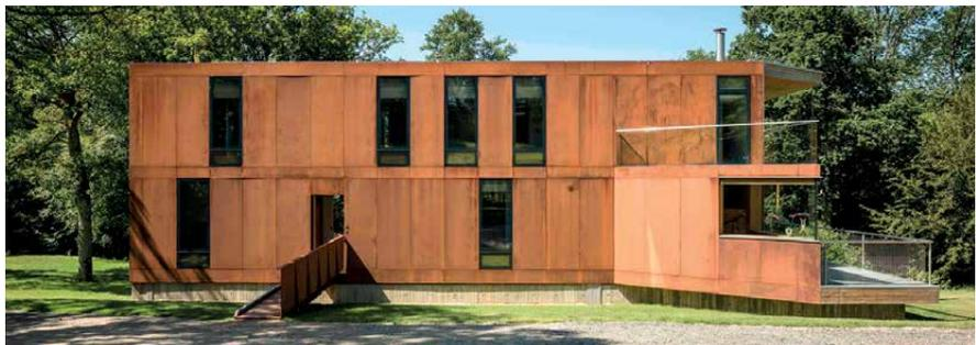
The use of structural steelwork enabled the 15m clear span to be achieved at the lower ground floor level swimming pool, while providing floor-to-ceiling openings to the upper floors on the same elevation.
