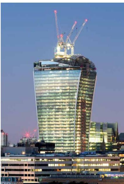
The north and south elevations of the structure have a fully glazed profile, while the east and west elevations feature vertical aluminium louvres for solar shading. The louvres line up with the steel members that make up the portal frames over the Sky Garden, creating the impression that they wrap over the building.
