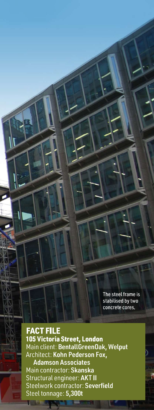
The steel design incorporates terraces on all of the upper floors.
