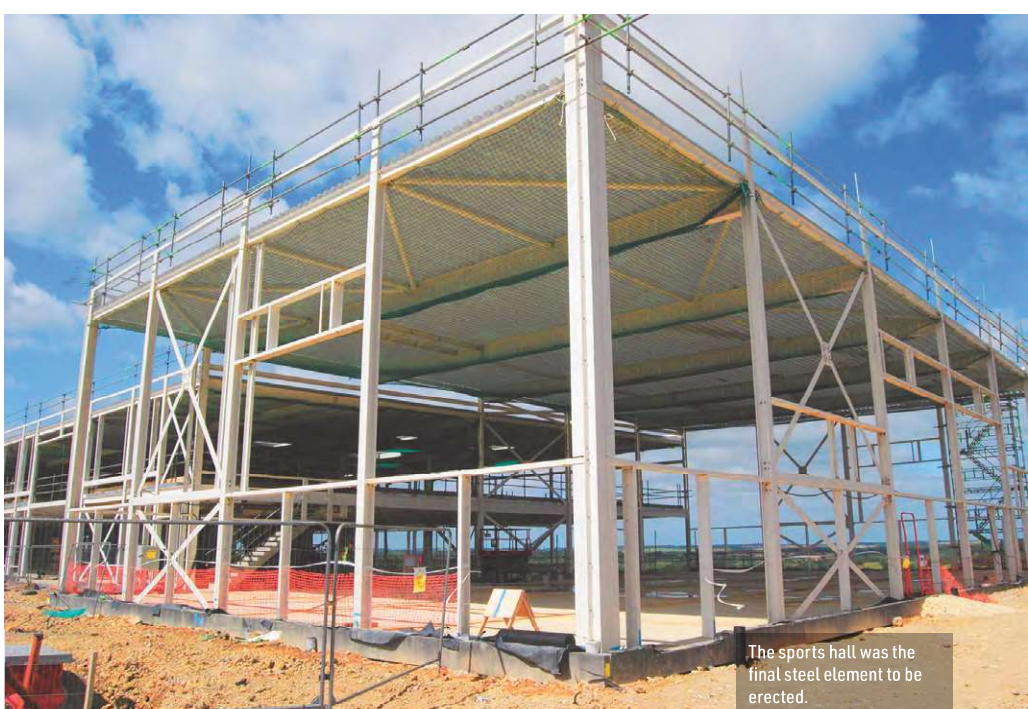
Cross bracings are located in and around stairwells.
