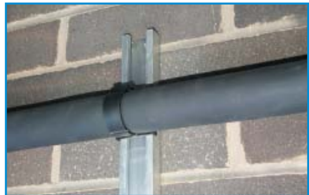
Figure 16: Polymer pipe clips are easy to release and re-locate, and are designed to clamp around insulation.
