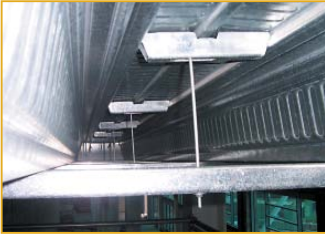
Figure 4: A Slimdek 2 wedge suspension hanger developed for the Corus SlimdekW system. ©Lindapter.
