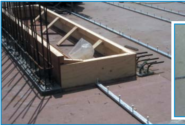
Left: figure 13: Halfen channel laid out prior to a concrete pour. Below, figure 14: A drop-rod fitted to the Halfen channel. Note the thermal insulation.
