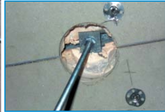
Left: figure 13: Halfen channel laid out prior to a concrete pour. Below, figure 14: A drop-rod fitted to the Halfen channel. Note the thermal insulation.
