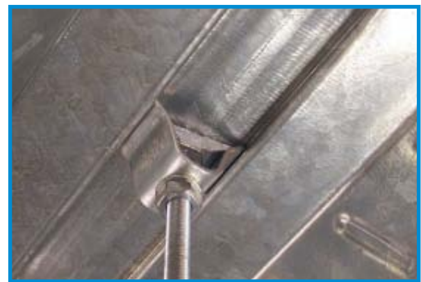
Figure 1: A wedge-nut system for fixing services to steel decking. ©Lindapter.
