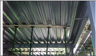
Normally, props are placed at either mid-span (one line of props) or at third points (2 lines of props) within a span. The decking sheets should never be interrupted (cut) at the location of a temporary support, and the decking should not be fastened to the temporary supports.
