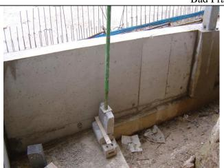
The decking layout drawings should show the extent and lines of temporary supports Bearing lengths are typically in the 75 to 100mm range.
