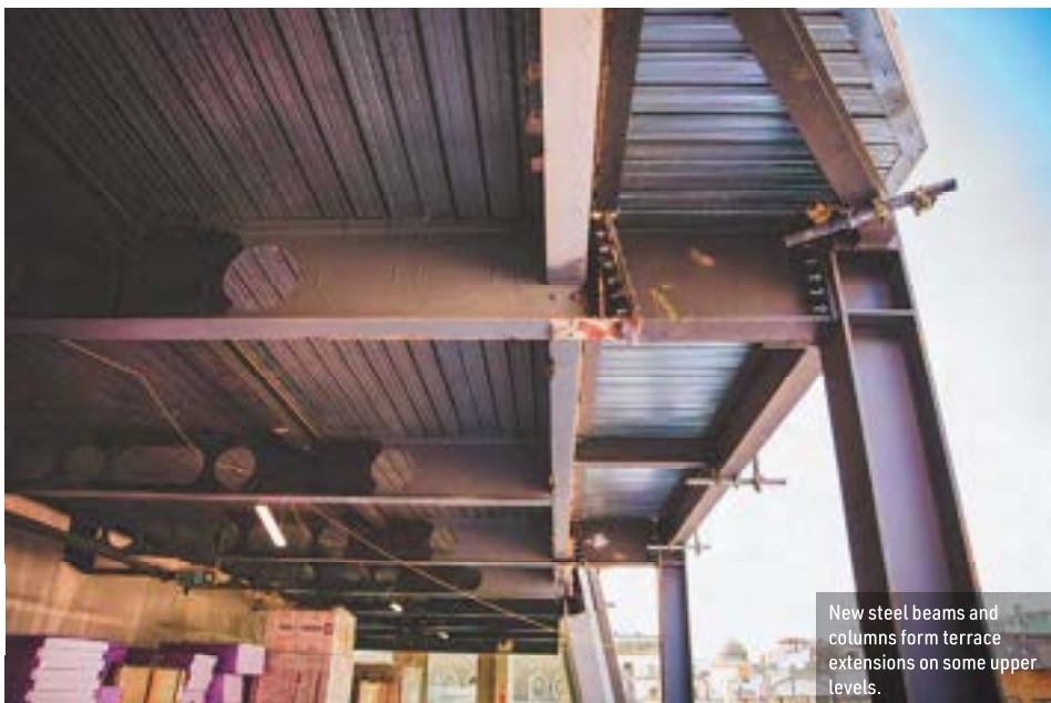
Two new steel-framed floors are being added to the building.
