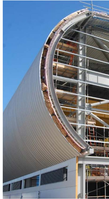
**A** steel-framed facilities building at the Harwell Science Campus has been designed to provide column-free testing and storage space, as well as to fit unobtrusively into the rural landscape.
