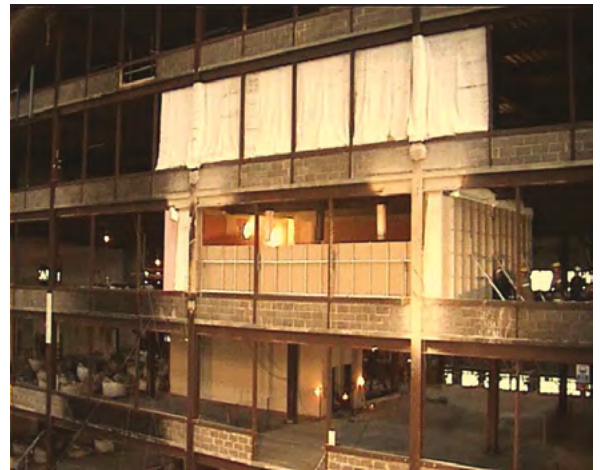
Steel framed building at Cardington - Fire test No.7
