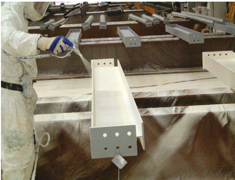
Application of intumescent paint. Courtesy of Severfield
