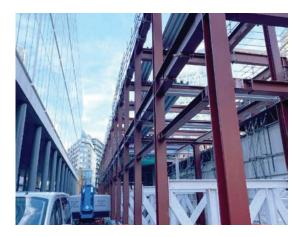
Several logistical challenges had to be managed during the construction of the steel frame, as the structure is situated above an existing basement vehicle ramp. The basement, which serves as a car park for an adjacent building, remained operational throughout the construction. Above ground, the site was very confined, with much of the available space taken up by the new building's footprint.
