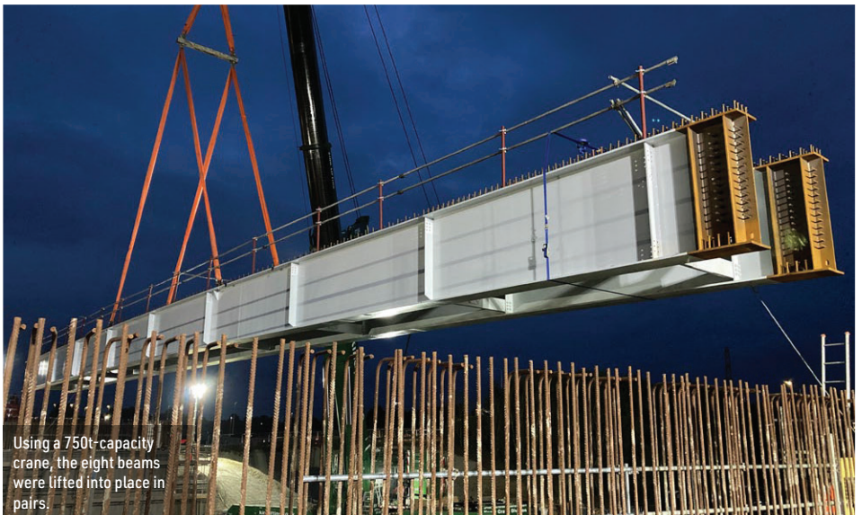
The bridge beams are long enough to accommodate extra traffic lanes if the A249 was to be upgraded.
