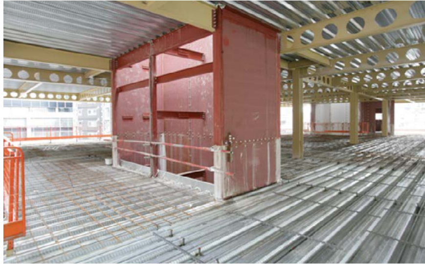
Figure 2.11 – Completed core and floor prior to concreting
