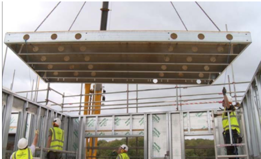
Figure 4.9 – Erection of a floor cassette
