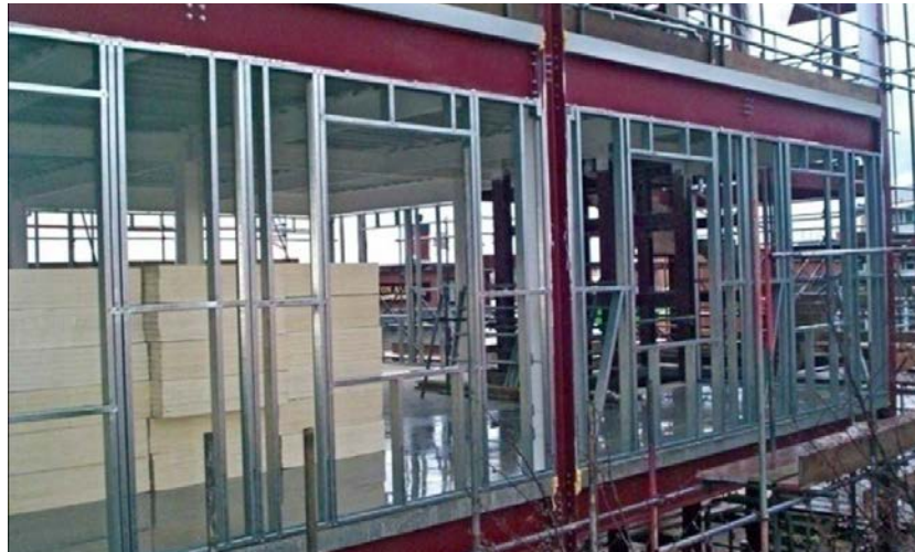
Figure 4.15 – Light steel infill wall used in a multi-storey steel-framed residential building (Image courtesy of Metek UK)
