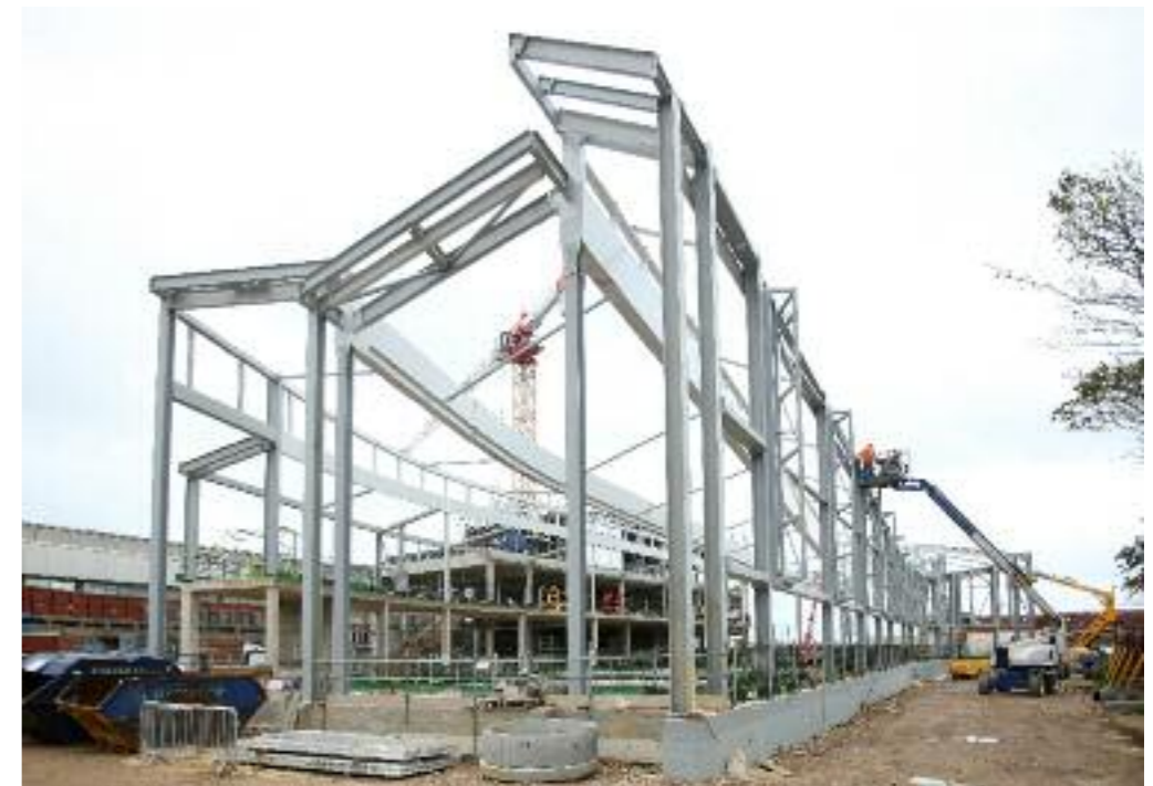
Left Steelwork moment frame model; software employed in the steelwork design included Nemetschek's Scia Engineer and Revit 3D (ph: AECOM).
