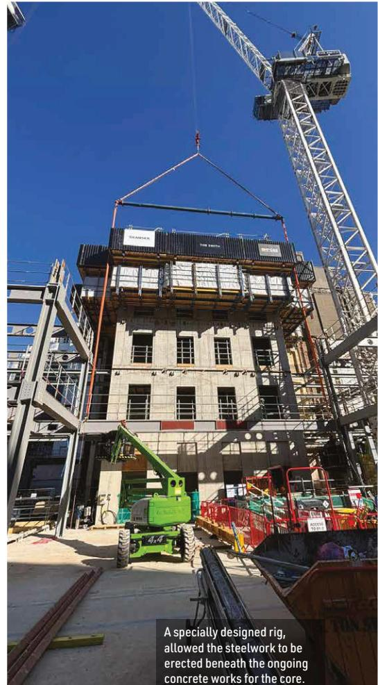
A specially designed rig, allowed the steelwork to be erected beneath the ongoing concrete works for the core.
