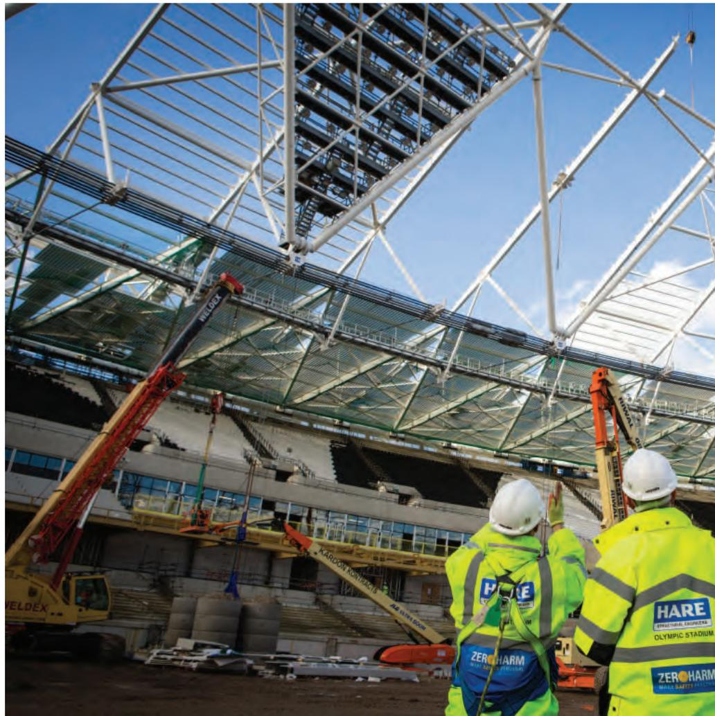
solution was a design where the steel cables carried most of the downward vertical loads, in similar fashion to a suspension bridge.
