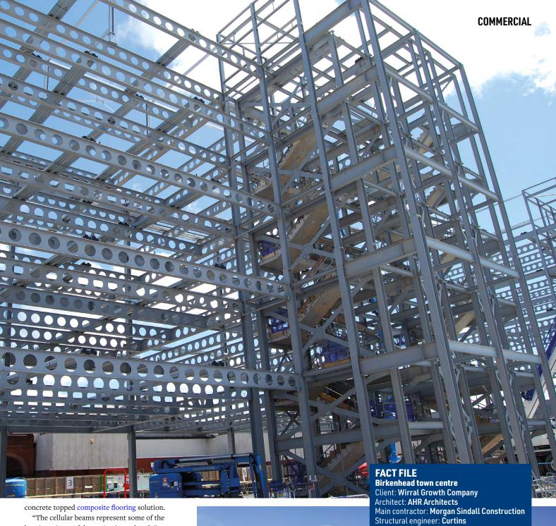
"The cellular beams represent some of the heaviest pieces of the project's steelwork," says Leach Structural Steelwork Site Supervisor Anthony May. "Although the majority are around 2.5t, some of the beams are up 6.5t each."
