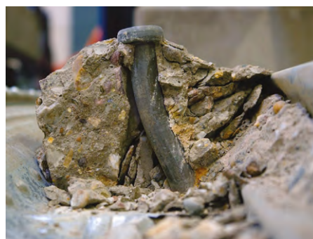
Figure 1: Deformation (slip) of a 19mm diameter shear stud in transverse decking at failure (courtesy University of Luxembourg)
