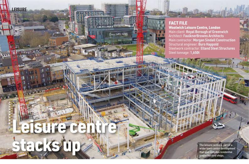
Aiming to achieve a BREEAM 'Outstanding' rating and set to be one of the UK's largest urban facilities, structural steelwork has provided the Woolwich Leisure Centre with the required efficient column-free design.
