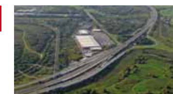
Repairs avoided a £100m viaduct rebuild.
