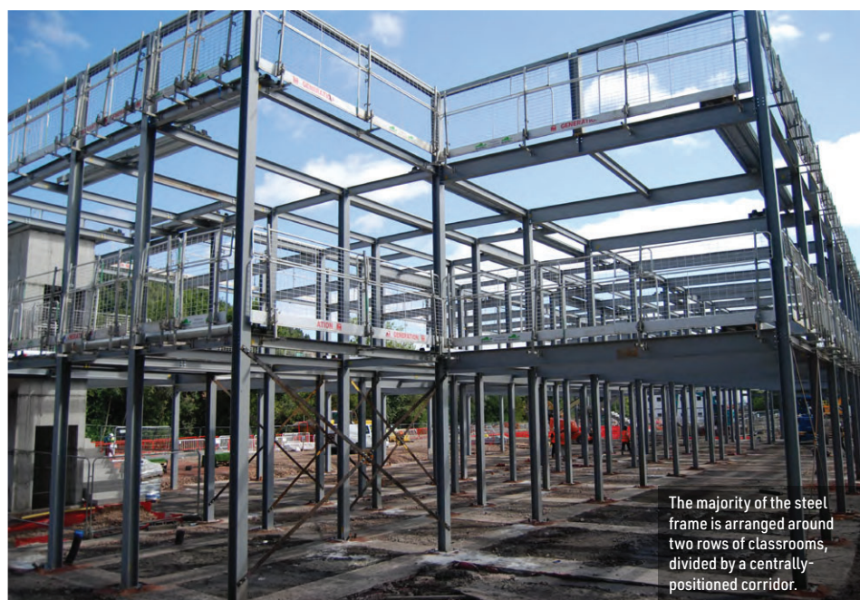
As part of its steel package, SSF also installed edge protection to the main frame.
