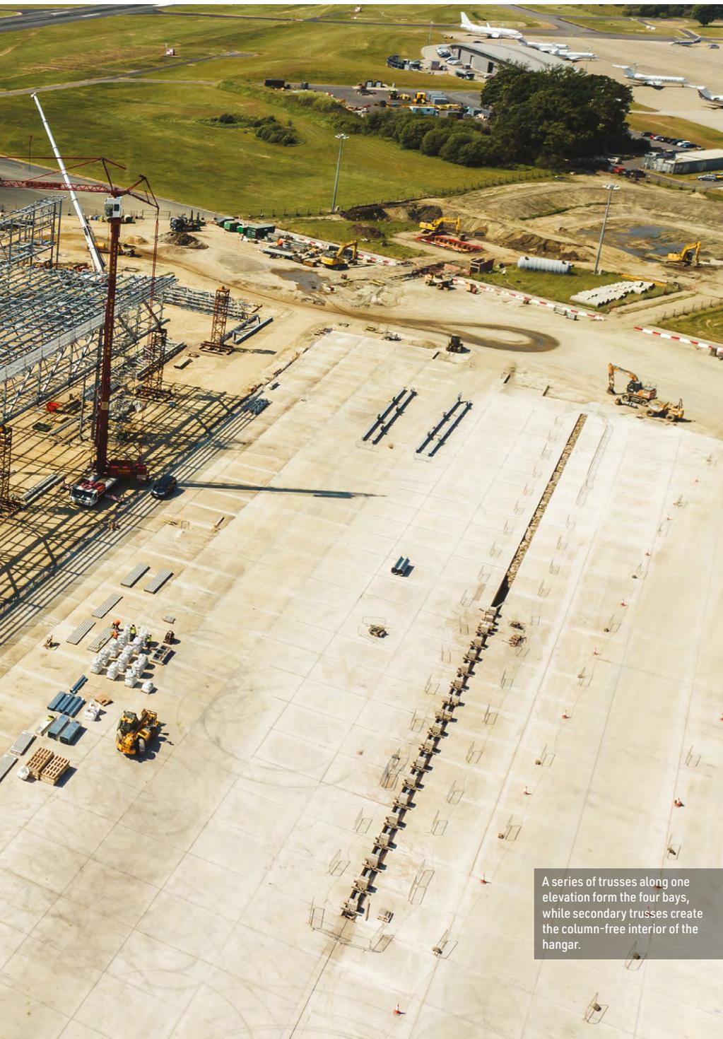
A series of trusses along one elevation form the four bays, while secondary trusses create the column-free interior of the hangar.
