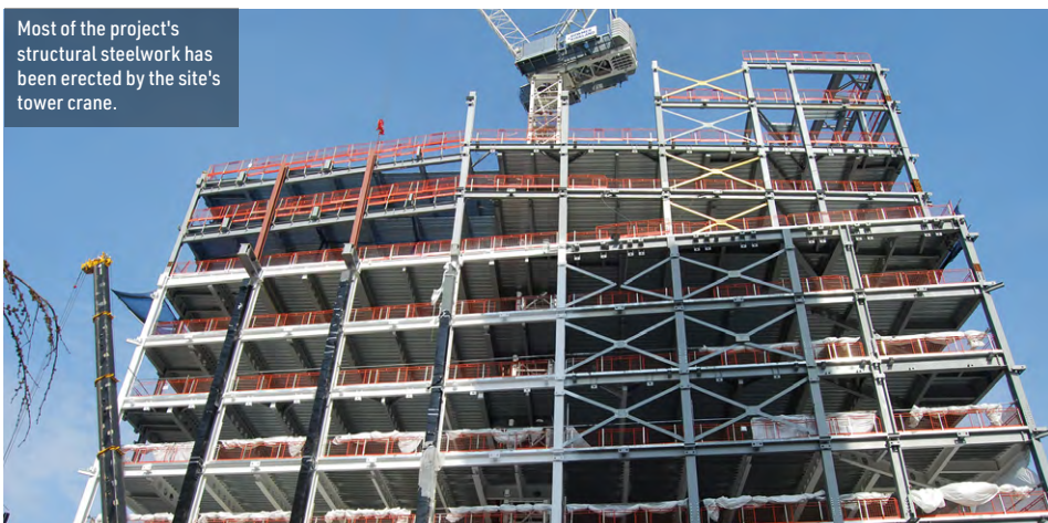
For ease of programme, the cantilevering steel elements are being erected once the cladding installation has reached level seven.
