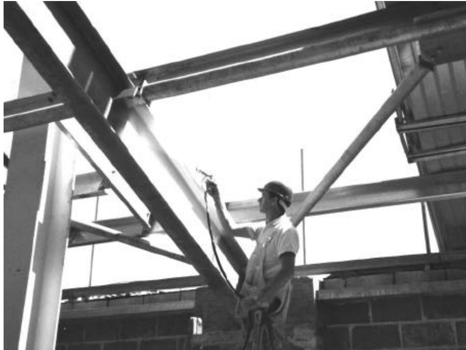
Figure 8.7 Thin film intumescent coating being applied
