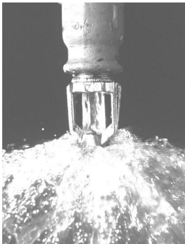
Figure 5.2 A sprinkler head in operation
