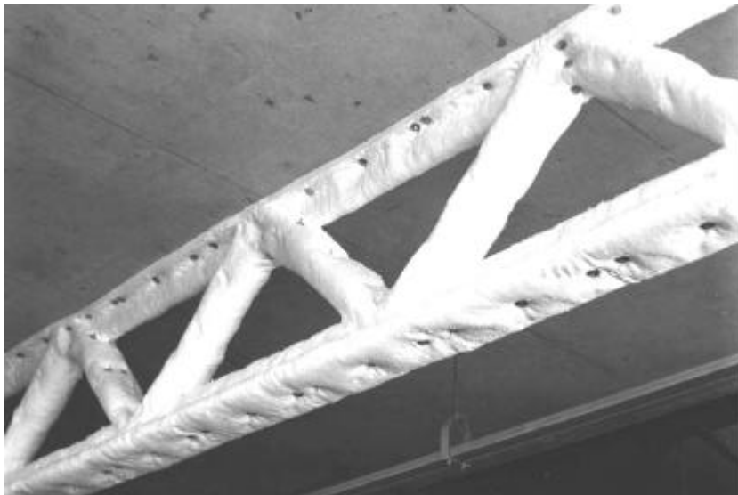
Figure 8.5 Pin-fixed blanket applied to truss
