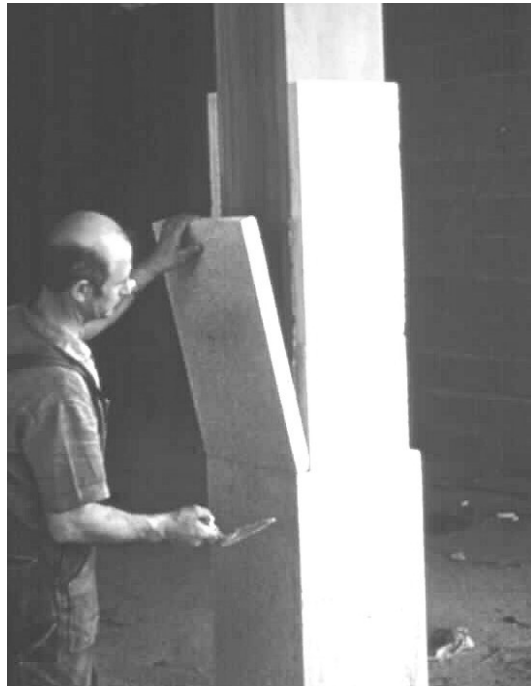
Figure 8.3 Board fire protection applied to a column
