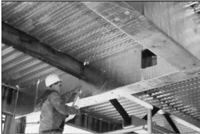
Figure 8.4 Foil covered fibre board applied to beams
