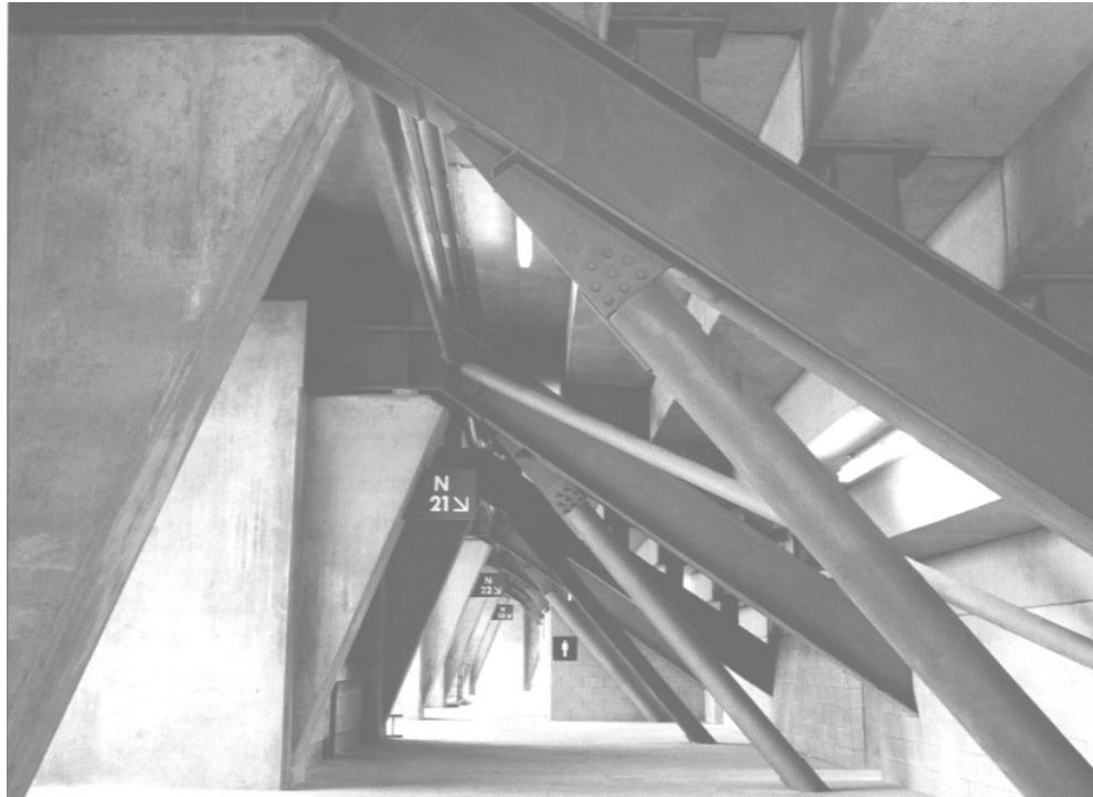
Figure 7.10 Unprotected steel beams supporting a grandstand
