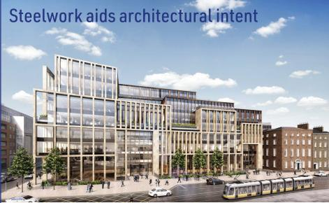
I S teel was chosen on this project to deal with a number of design considerations. The first was programme, and the benefit with steel lies in the capacity for manufacture off site. This, coupled with a very swift erection process, made steel a more desirable option than a concrete frame," explains Henry J. Lyons Associate Amy Murphy.
