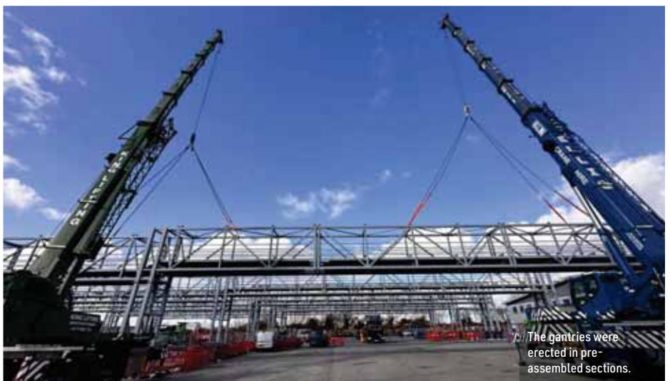
The gantries are supported by braced column towers.
