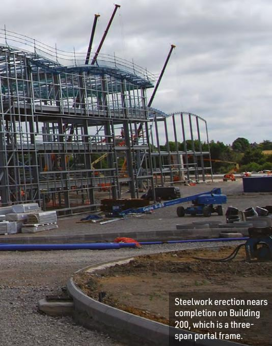
Steelwork erection nears completion on Building 200, which is a three-span portal frame.
