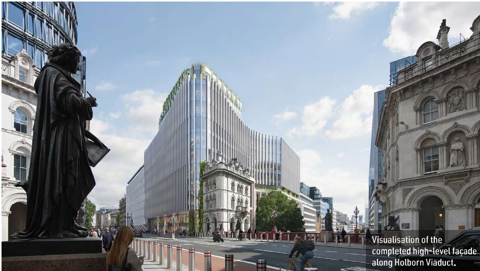
From the fourth floor upwards, the building has cantilevers along the Holborn Viaduct elevation.
