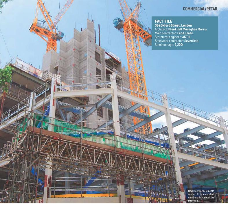
beams supporting poured in-situ concrete floors, completed the core construction.
