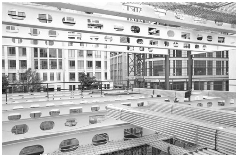
Figure 4.9 Fabricated beam with off-site fire protection
