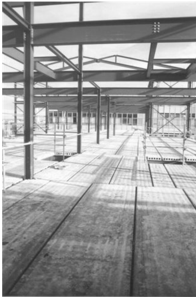
Figure 4.17 Precast concrete units on steelwork
