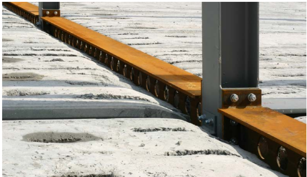
Figure 4.7 Shallow floor beam and precast planks
