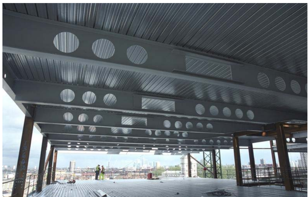
Figure 4.3 Long span composite beams providing column-free space
