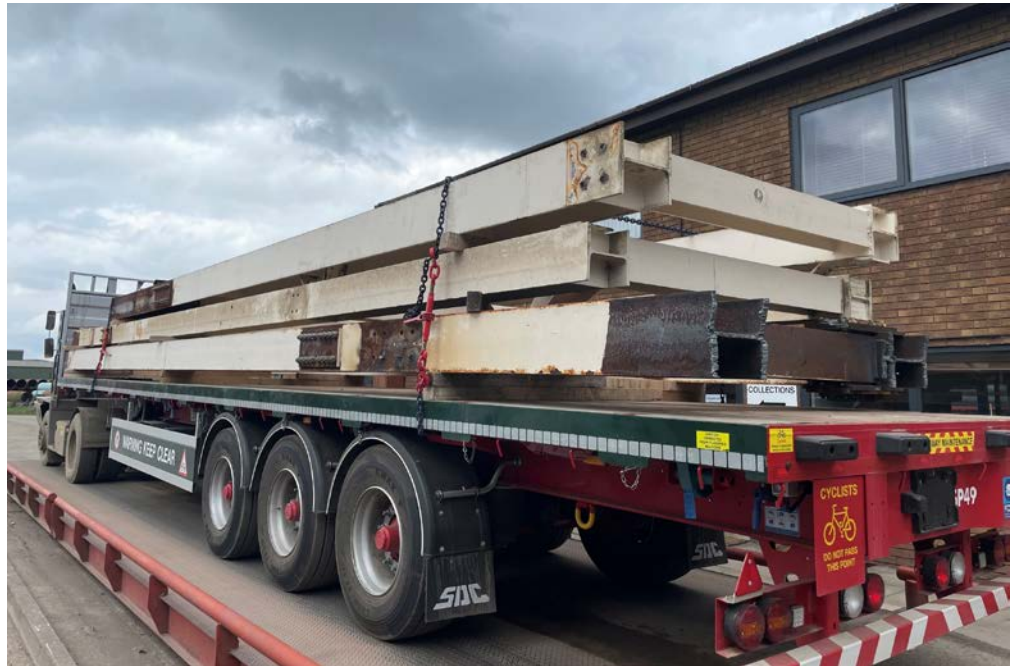
Figure 3.3 Recovered structural steelwork
