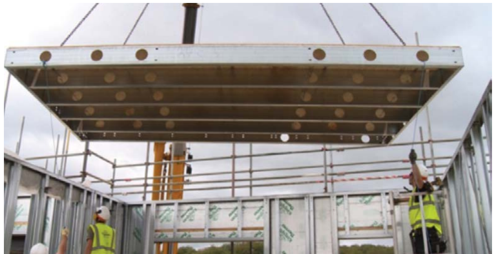
Figure 10.3 Light gauge steel floor cassette
