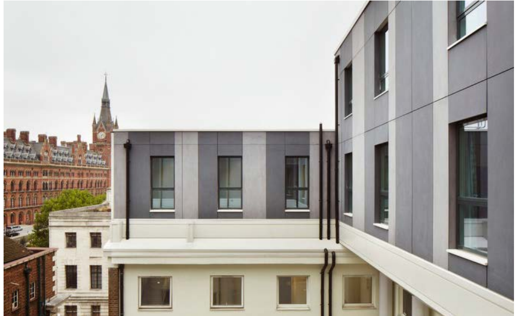
Figure 3.2 Light gauge modular roof top development
