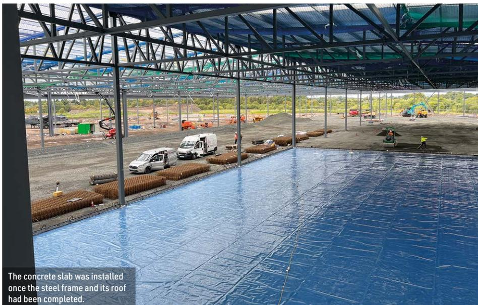
The concrete slab was installed once the steel frame and its roof had been completed.
