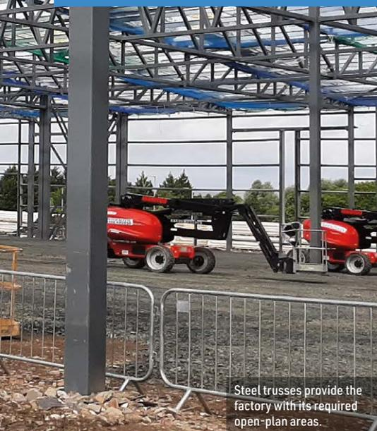
Steel trusses provide the factory with its required open-plan areas.
