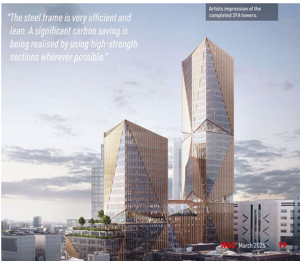
The project is characterised by saw-toothed steel-framed facades.
