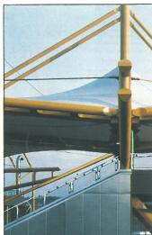
raking support member beneath the terraced seating and linking these two members at spectator level by a beam which would then also support the concourse floor, a tied A frame was generated to solve these apparently conflicting ideals. The roof columns were continued down through the A frame to provide transverse stability above its apex and also to act in tension to provide a midspan support to the tie beam.
