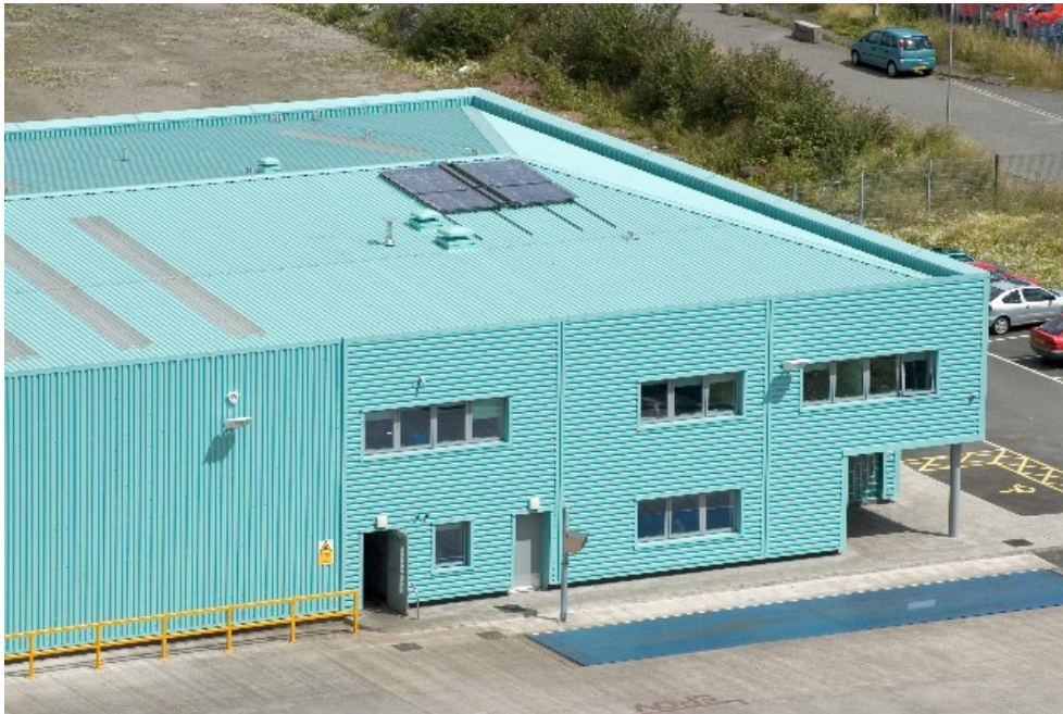
Figure 2.10 Build-up roofing system with internal gutters hidden behind the parapet wall (Photograph by kind permission of Corus Colors)
