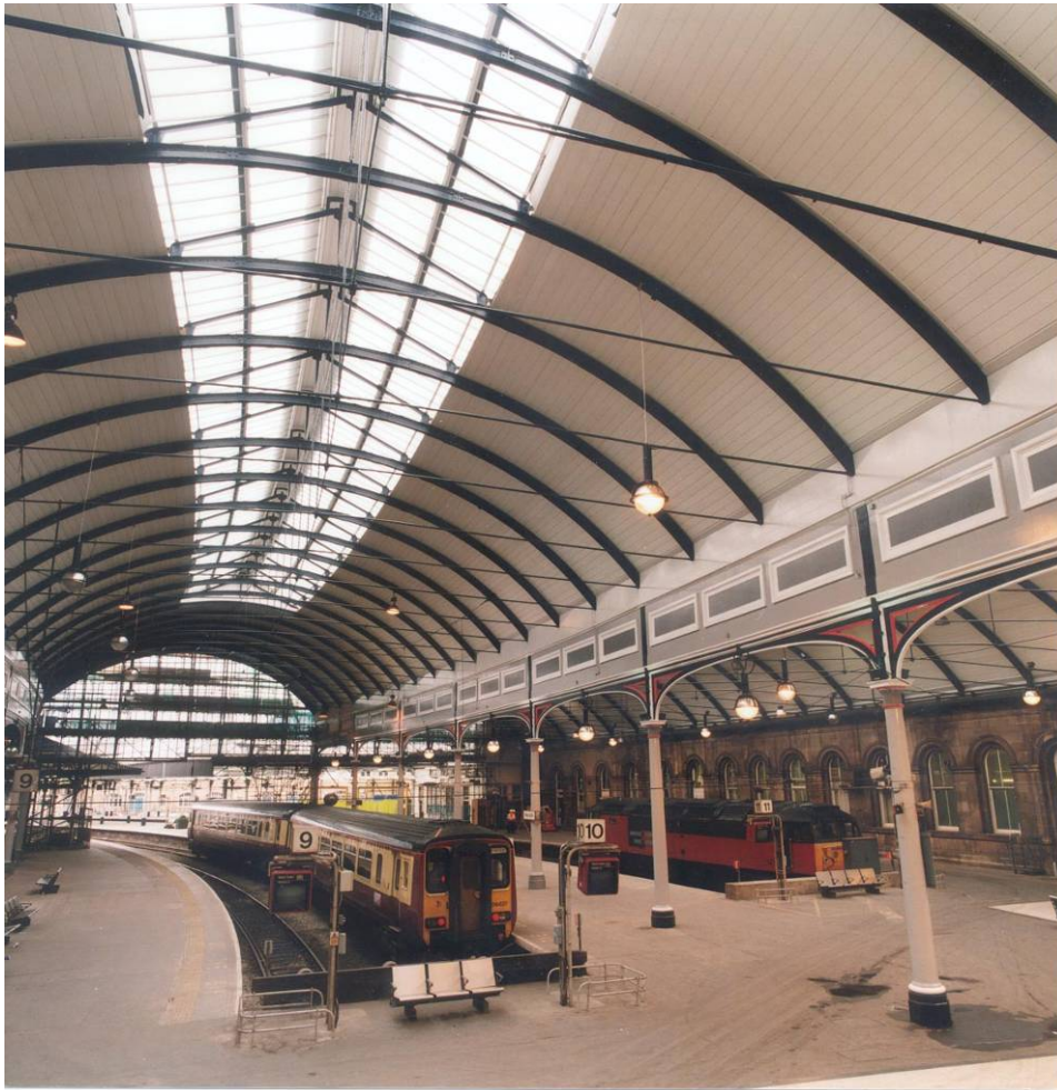
Figure 2.2 Bright white pressed liner profile have been used on the refurbishment of the roof at Newcastle Station to create the effects of timber planks (Photograph by kind permission of Corus Profiles & Panels)
