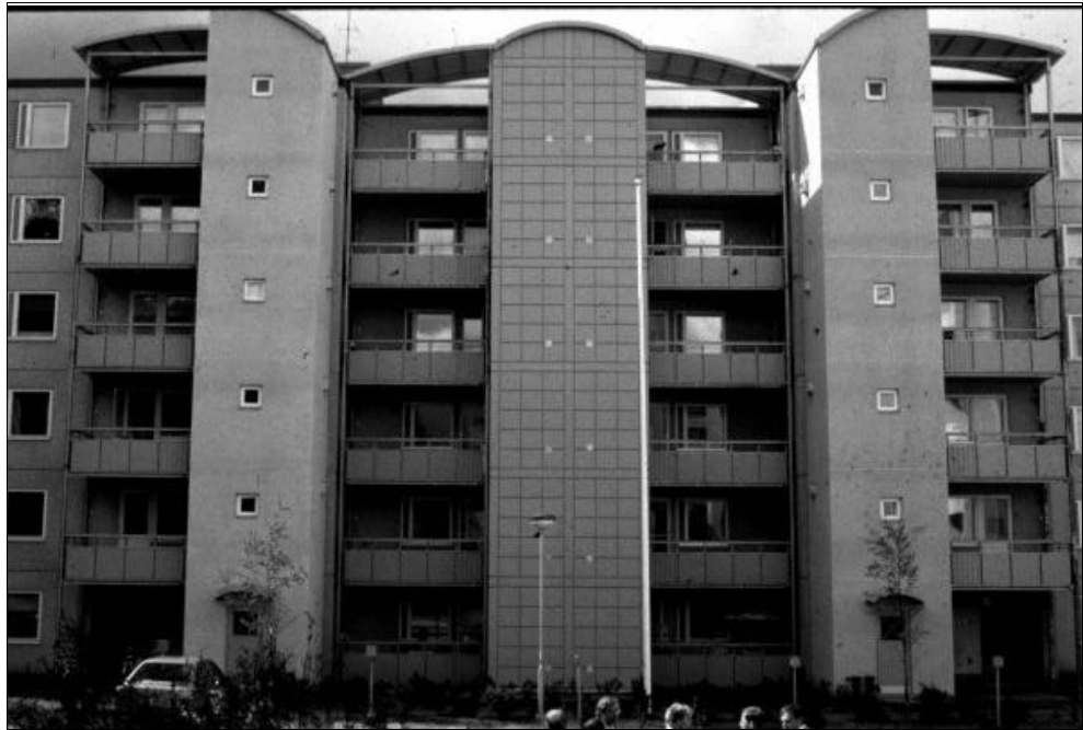
Figure 11.2 Completed over-clad building in Forssa, Finland
