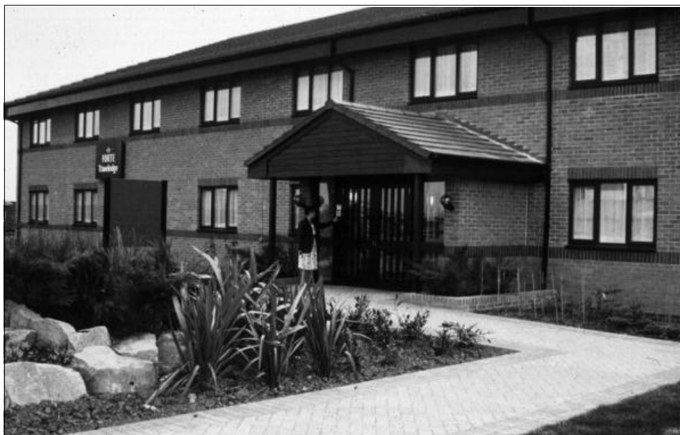
Figure 5.4 Terrapin Prospex system used for hotel construction
