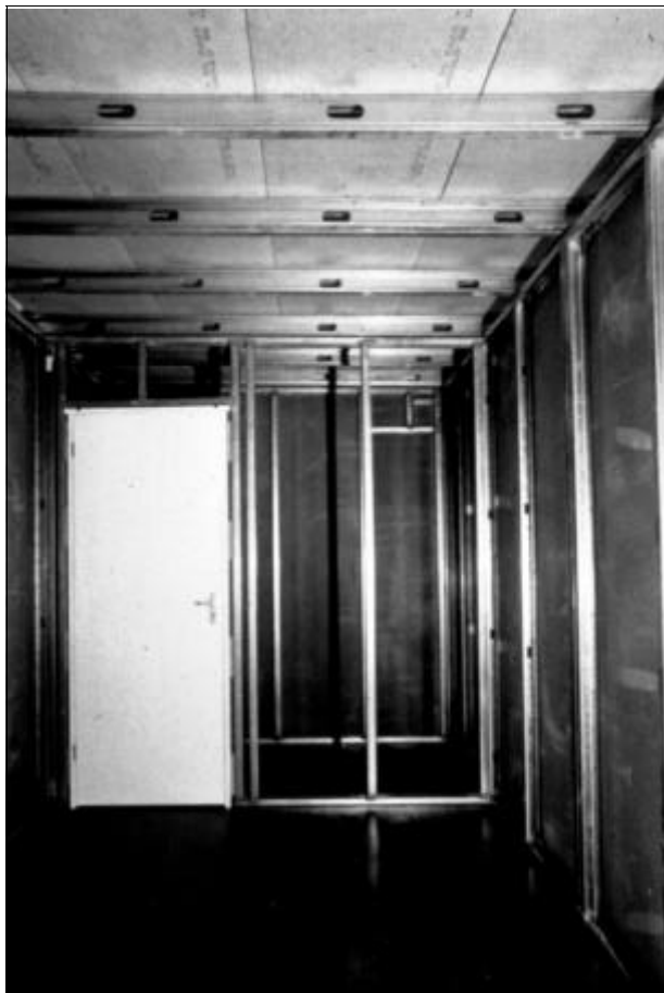
Figure 5.5 View inside modular bedroom before lining and fitting out
