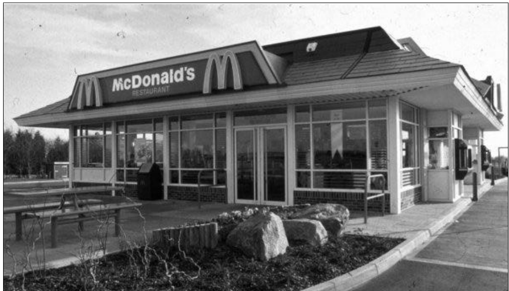
Figure 1.3 Fast-food restaurant, which is fitted out before delivery to site
