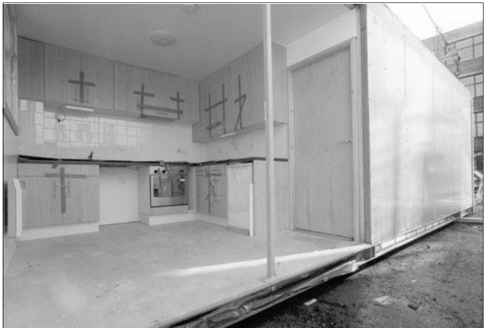
Figure 5.8 Internal view of kitchen module (temporary prop is removed after installation)
