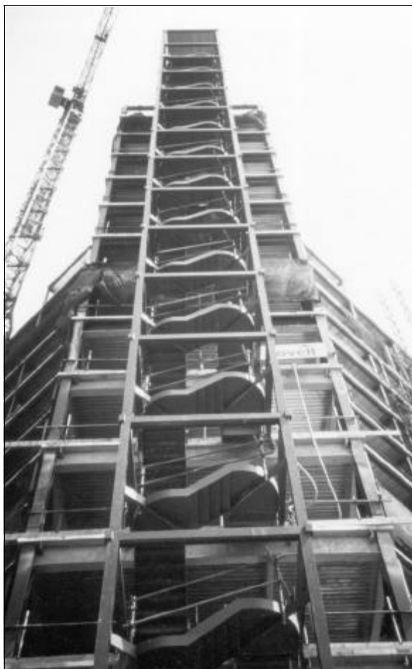
Figure 2.6 Prefabricated steel stairs used in a commercial building
