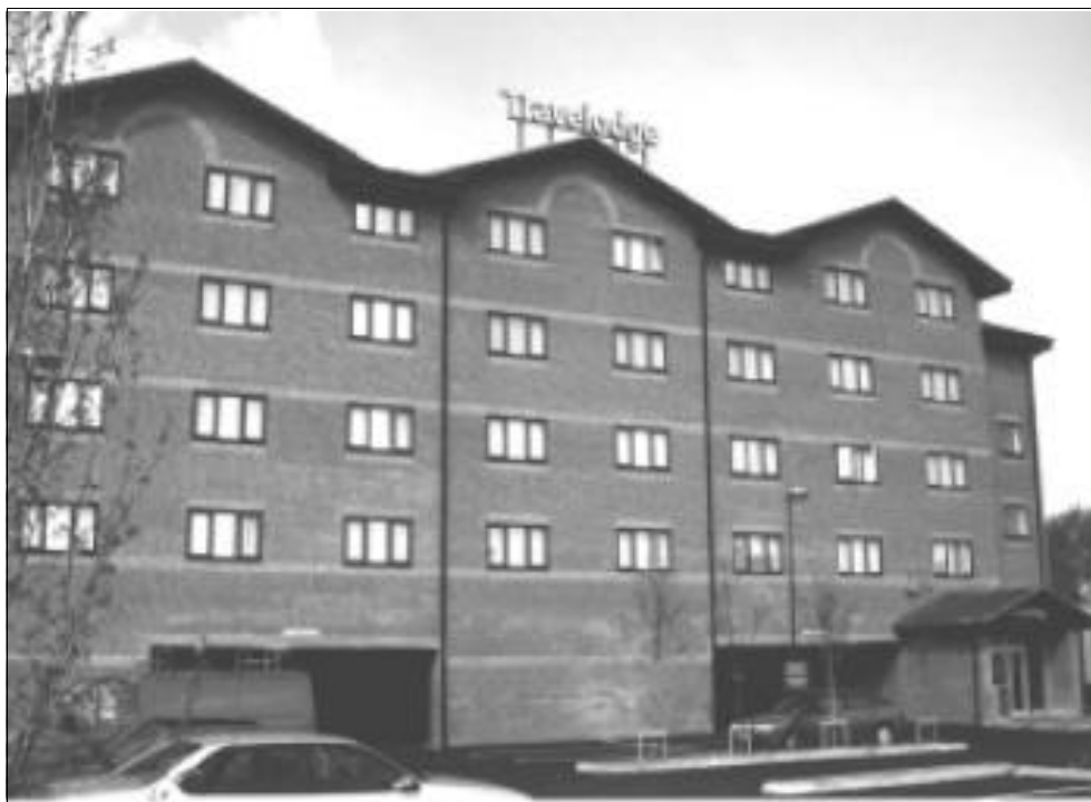
Figure 3.1 Multi-storey hotel using modular units
