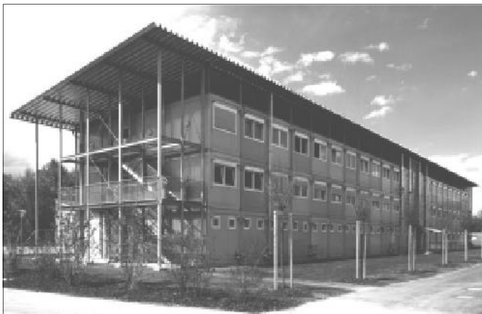
Figure 4.6 Modular office building in Munich
