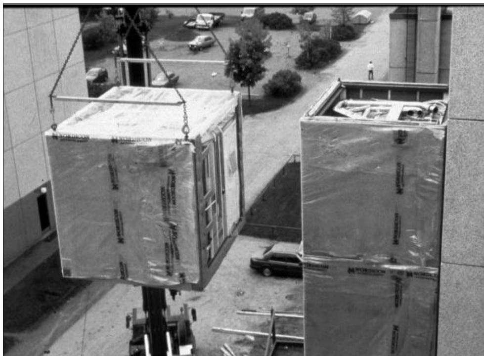
Figure 11.1 Installation of modular toilet units
