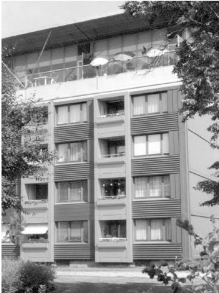
Figure 4.4 Renovation by over-cladding and modular roof-top extension in Denmark
