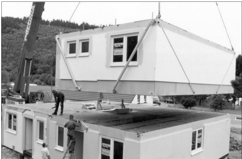
Figure 4.5 Modular unit for housing manufactured by Alho in Germany
