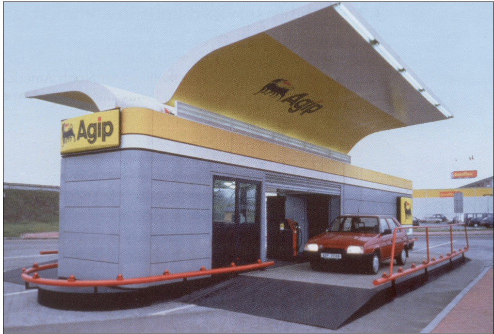
Figure 3.5 Portable petrol station and canopy
