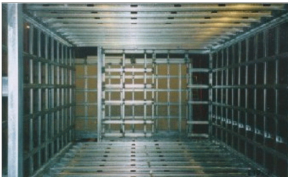
Figure 5.1 AyrFrame modules (unclad and unfinished at this stage)
