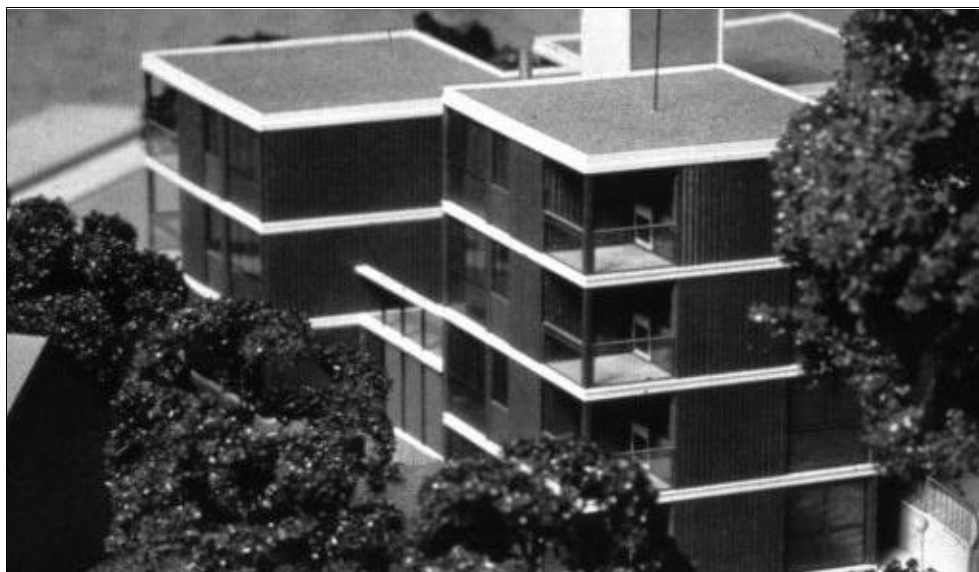
Figure 2.3 Early use of modular units in housing in the UK
