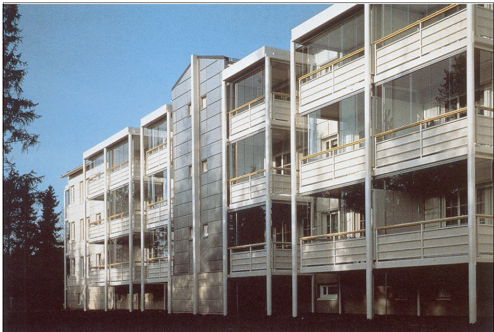
Figure 11.3 Completed over-clad building in Raahe, Finland
