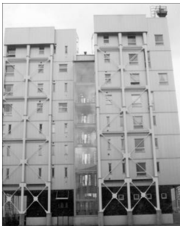
Figure 4.2 Modular units used in tubular framework in Tampere, Finland
