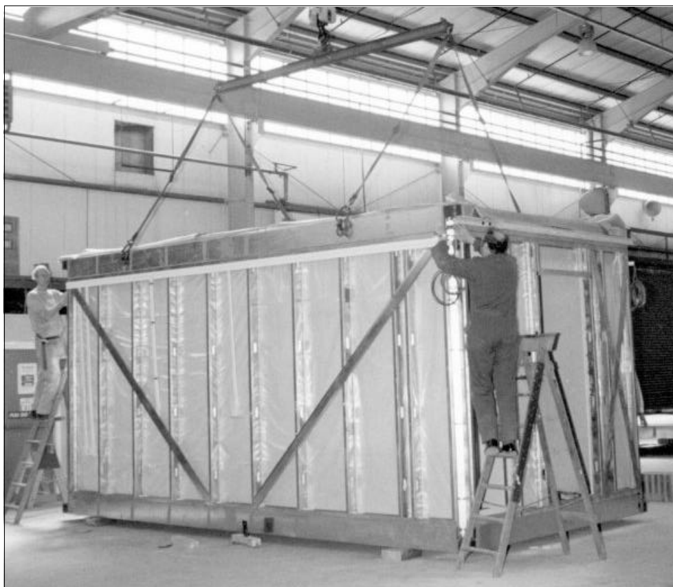
Figure 1.6 Light steel frame used in modular construction
