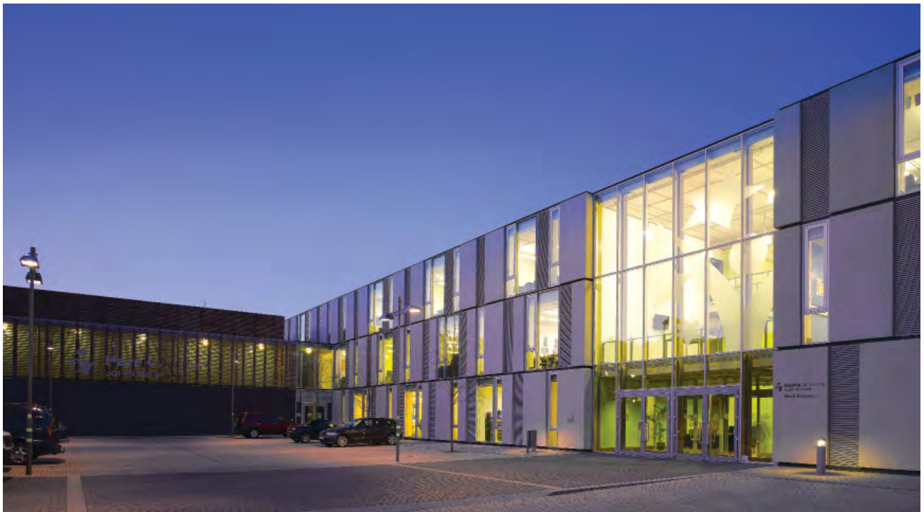
HARRIS ACADEMY, SOUTH NORWOOD, CROYDON
