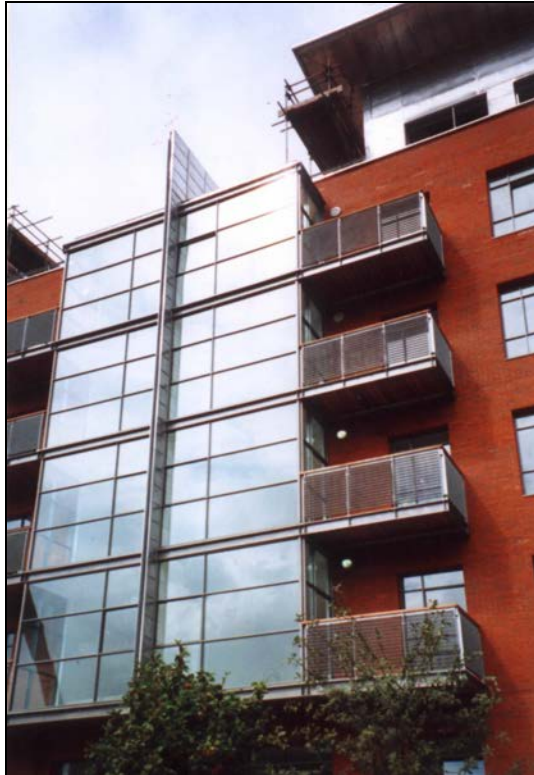
Figure 6.3 Cantilever balconies in a composite structure, Deansgate Quay, Manchester (Courtesy of Stephenson Bell)
