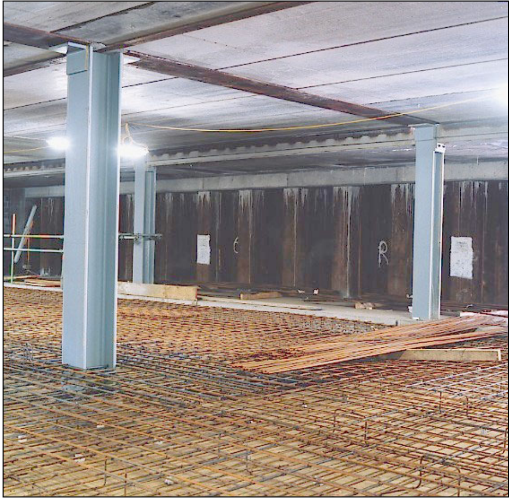
Figure 7.3 Use of Slimflor beams in basement construction
