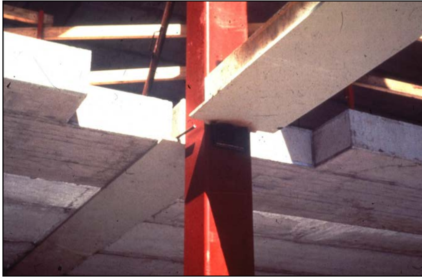
Figure 4.7 Slimflor beams supporting precast concrete slabs
