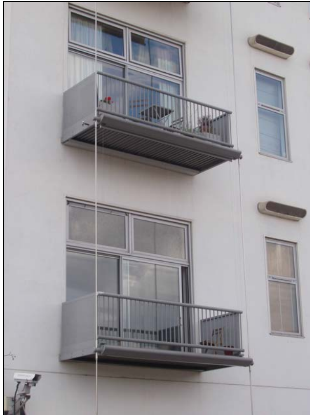
Figure 6.7 Suspended balconies (Piper Building, Fulham)
