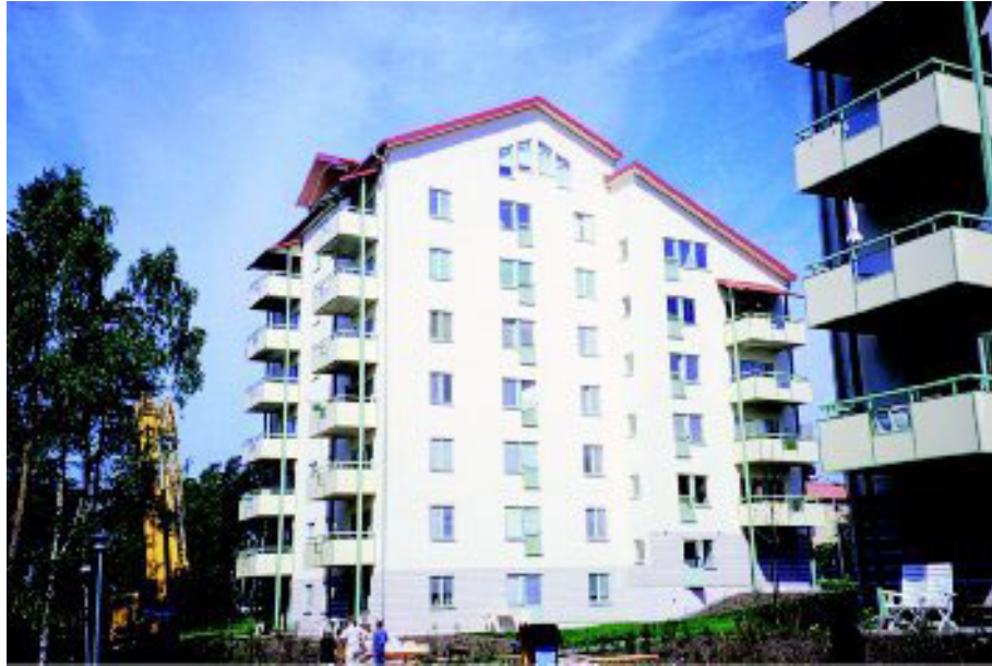
Figure 6.1 Stacked modular balconies (project in Sweden)
