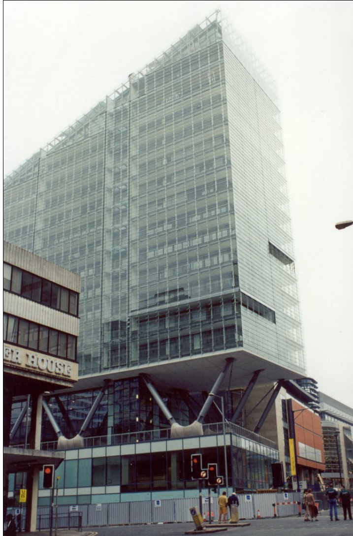
Figure 1.3 16-storey composite steel framed building in Manchester
