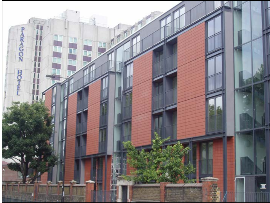
Figure 5.7 Clay tiled façade in a social housing project in Fulham
