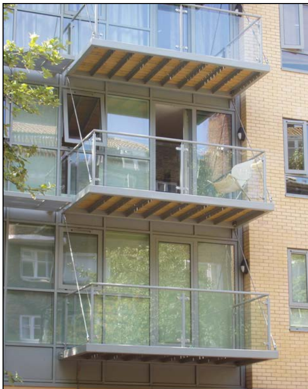
Figure 6.6 Tied balconies St Edmunds Terrace, Primrose Hill, London (Courtesy of HTA Architects)
