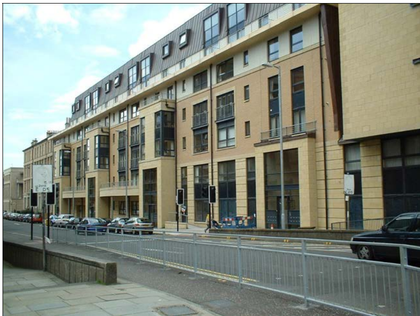
Figure 1.2 Variety of façade treatments in a steel framed residential building in Glasgow
