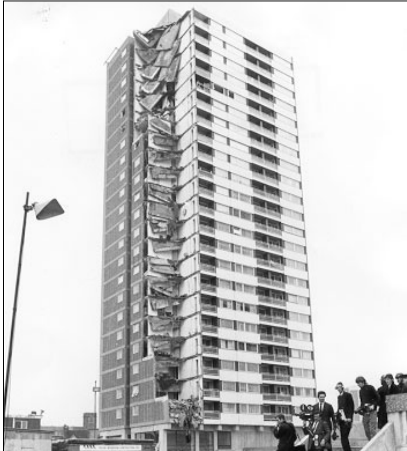
Figure 3.3 Partial collapse of a precast concrete structure dueto a gas explosion (Ronan Point)
