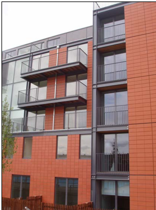
Figure 6.4 Cantilever and integral balconies at Beaufort Court, Fulham (Courtesy of Feilden Clegg Bradley)
