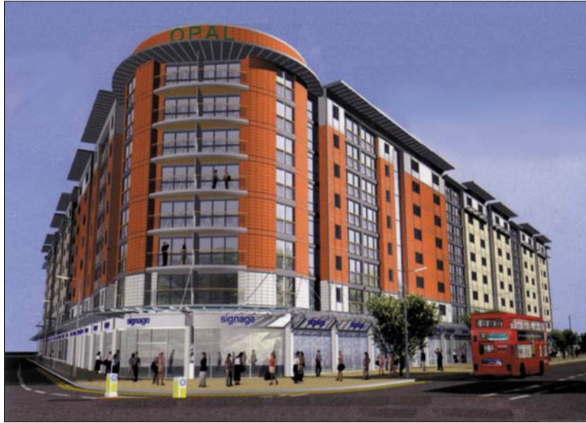
Figure 1.4 Eight-storey modular building in Manchester, supported on a composite frame at podium level
