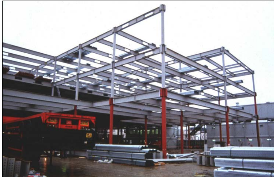
Figure 4.2 Long-span composite beams used in a multi-storey building
