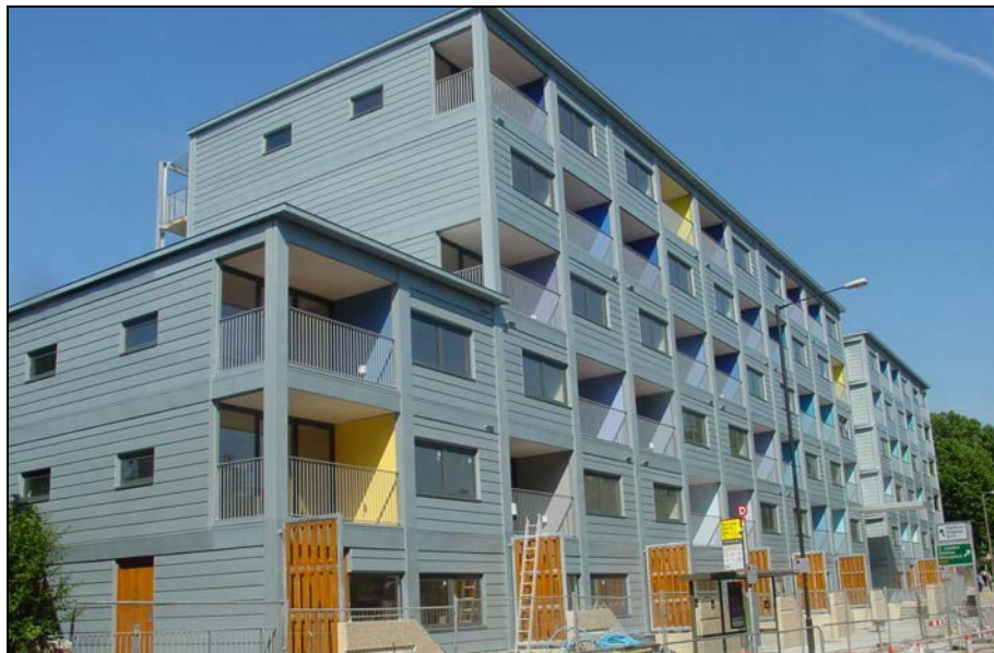
Figure 5.11 Zinc sheets used at Raines Court, London
