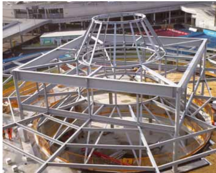
A steel and glass 'lantern' structure rises from level five of the civic drum
