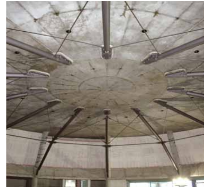
The community hall roof steelwork is finished with an intumescent coating
