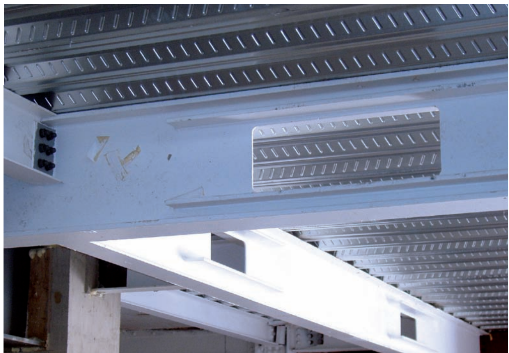
Figure 1.1 Isolated rectangular openings in a composite beam
