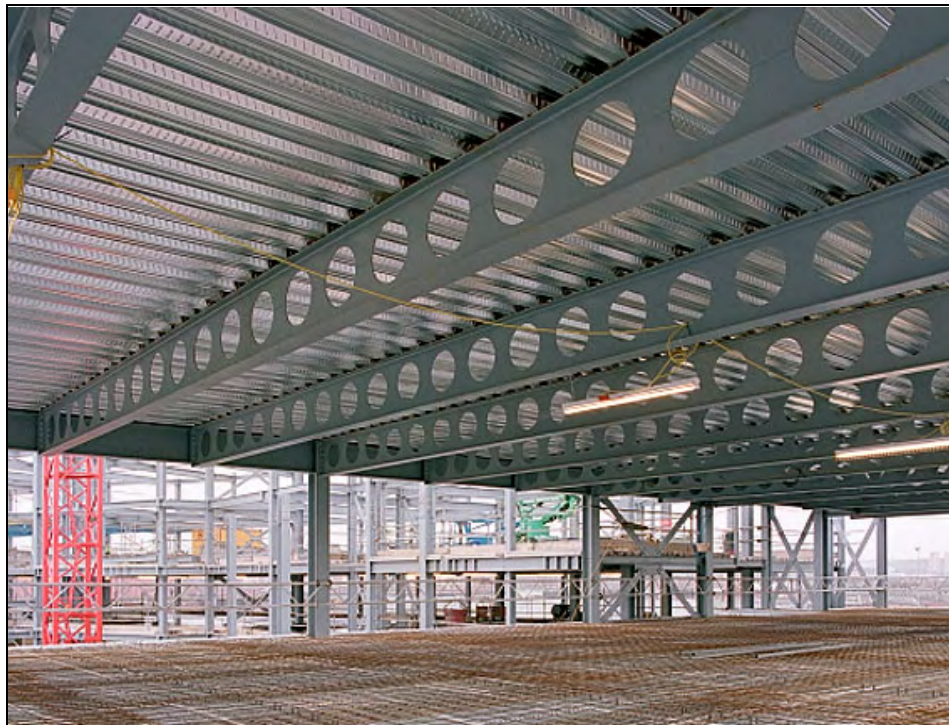
Figure 2.2 Long-span secondary beams with regular circular openings
