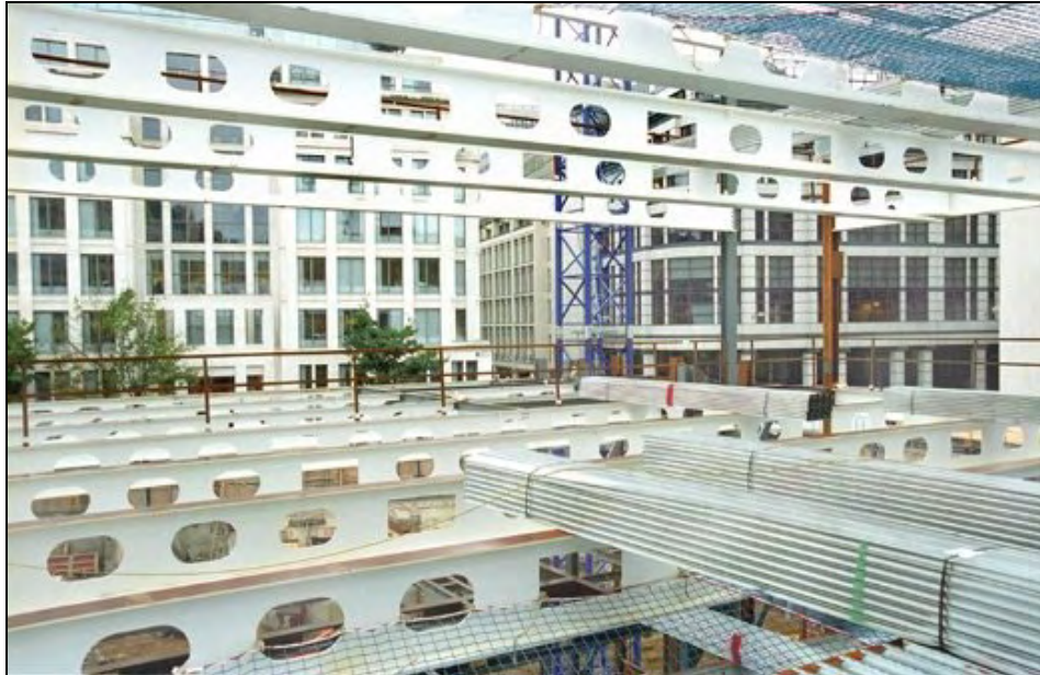
Figure 2.3 Fabricated beams with off-site fire protection
