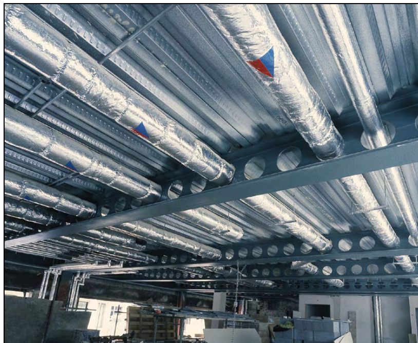
Figure 4.3 Cellular beams with circular ducting
