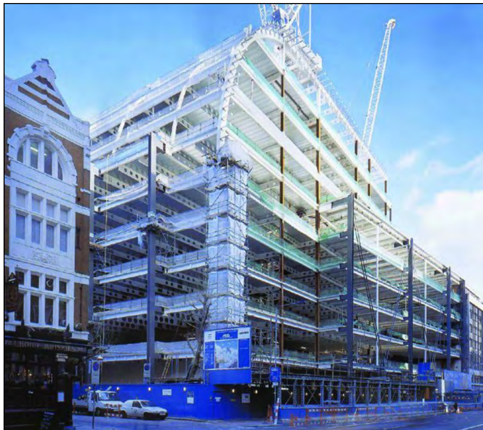
Figure 1.1 Long-span steel construction used at Mid City Place, London
