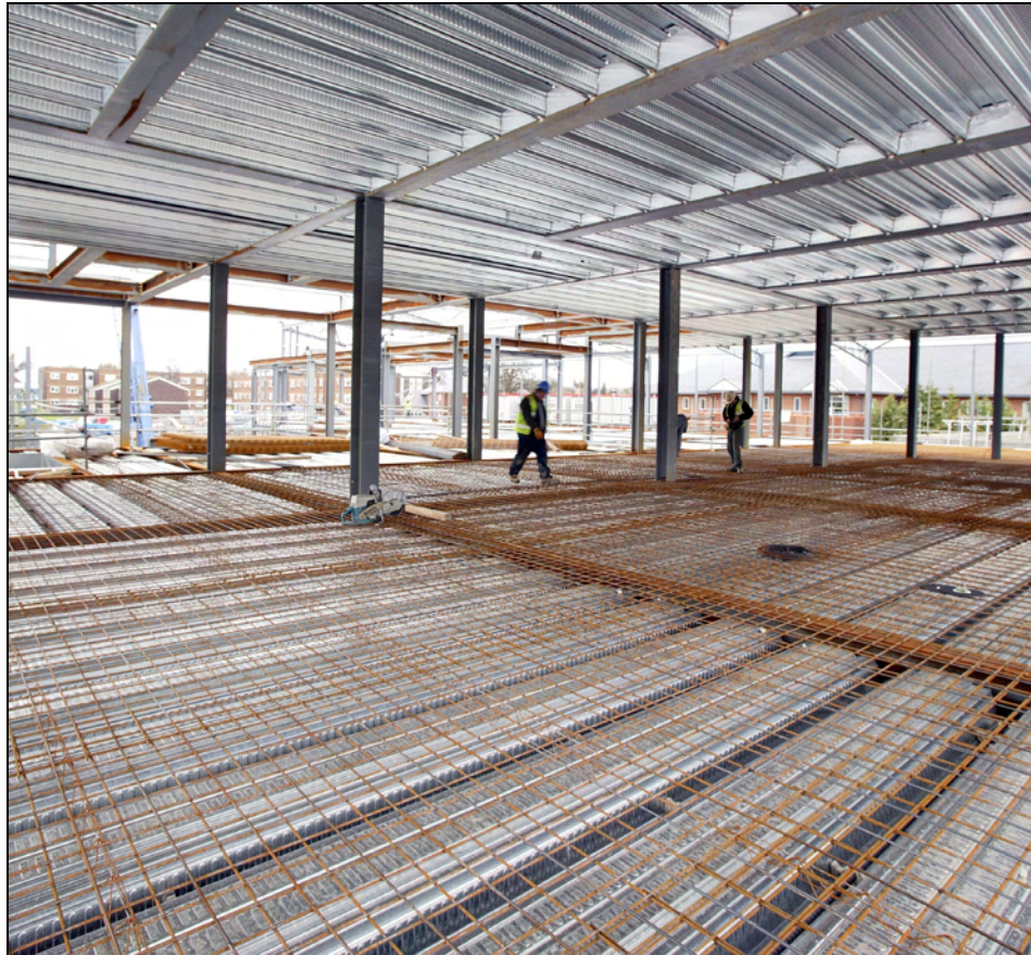
Figure 2.1 ASB sections and deep decking
