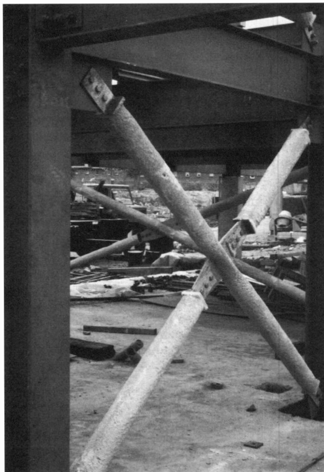
Figure 12.3 Fire protection to bracing members
