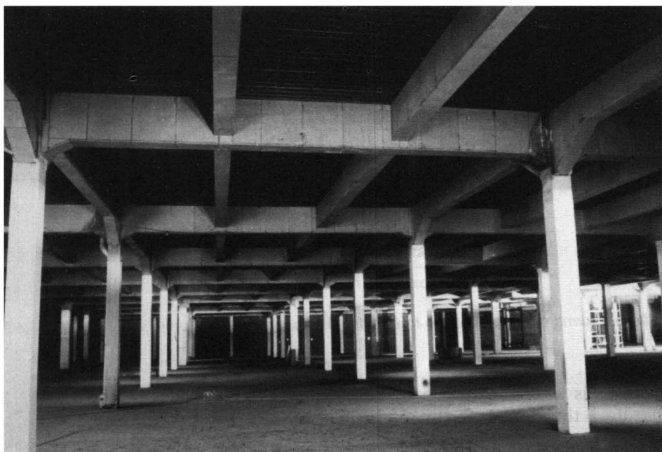
Figure 4.3 Box fire protection to steel members
