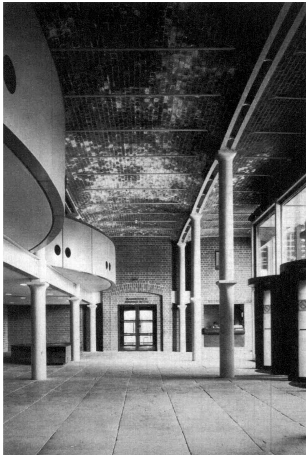
Figure 8.4 Intumescent paint protection to cast iron columns and beams
