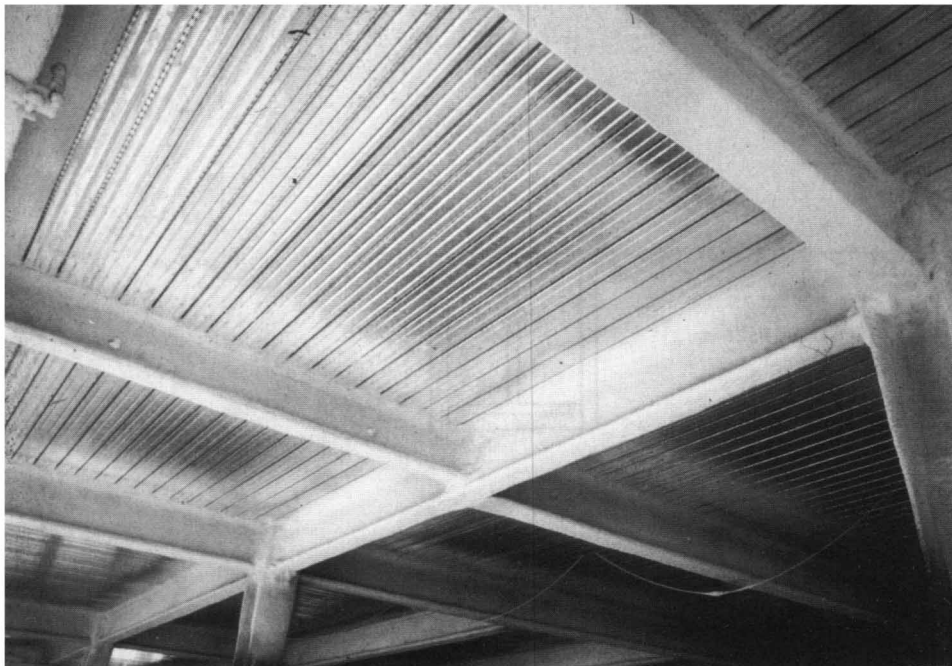
Figure 4.2 Profile fire protection to steel members
