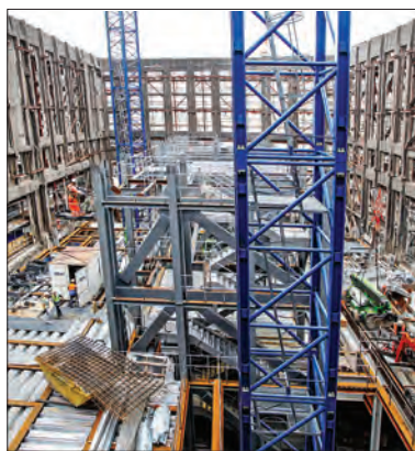
Top right: The feature roof frame will support a lightweight aluminium frame and glazing
