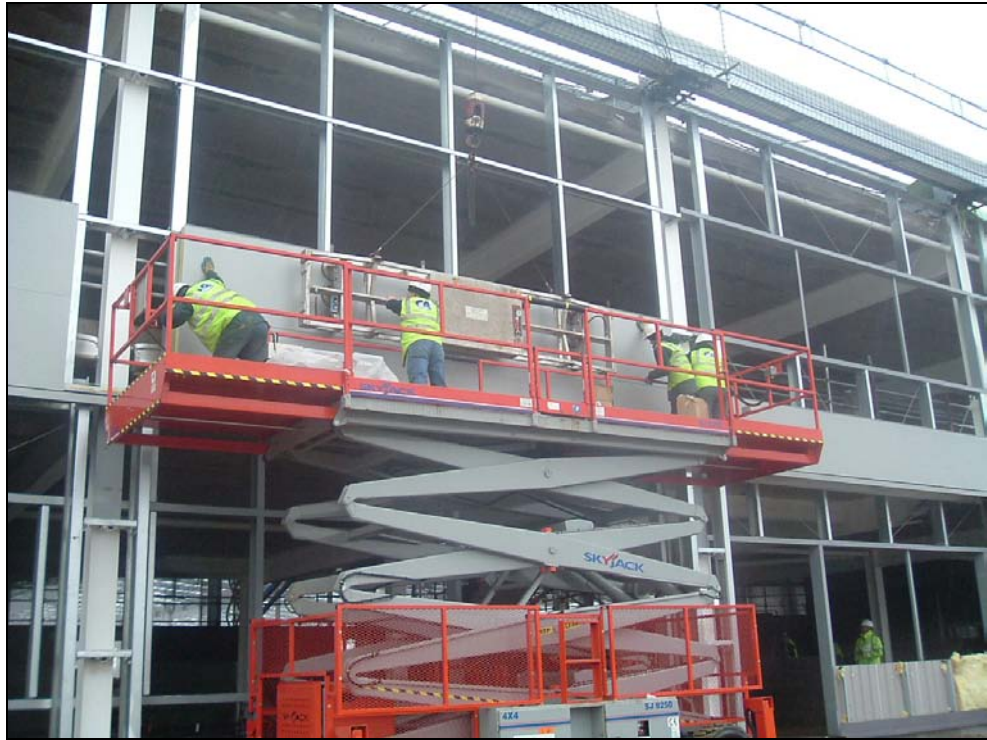
Figure 5.2 Wall cladding installation (Image courtesy of C A Roofing)
