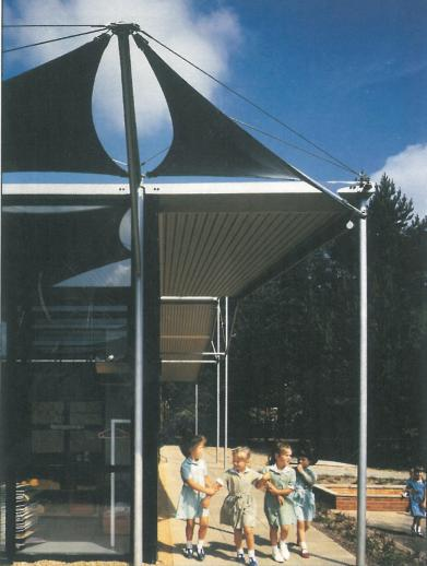
These frames are held both vertically and longitudinally by additional 2 metre deep cross-bracing members at right angles, reducing the effective height of the central columns and similarly reducing the size of the section used. At the eaves, a 90mm deep steel channel spans between the dumbells as a structural gutter, with the inner 76mm diameter CHS of the dumbell acting as the downpipe.
