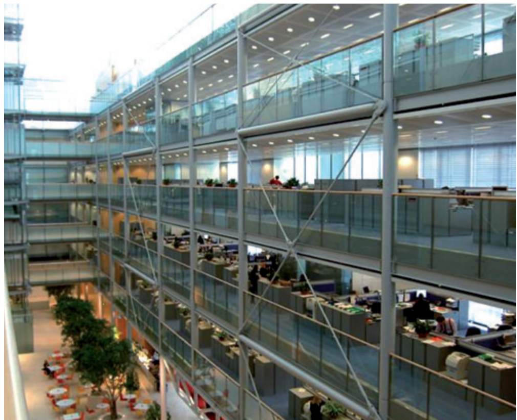
Figure 8.1 Concrete filled hollow section composite columns at the Wellcome Trust
