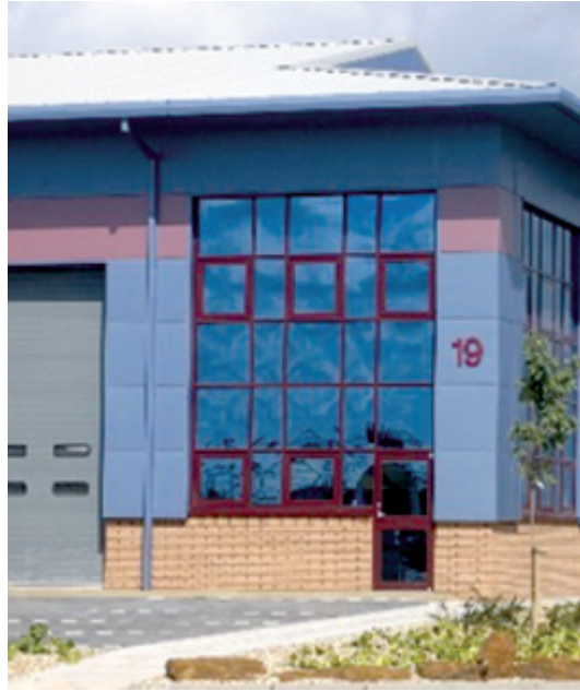
Figure 2.15 (Left) Large windows and use of composite panels with dado brick wall
