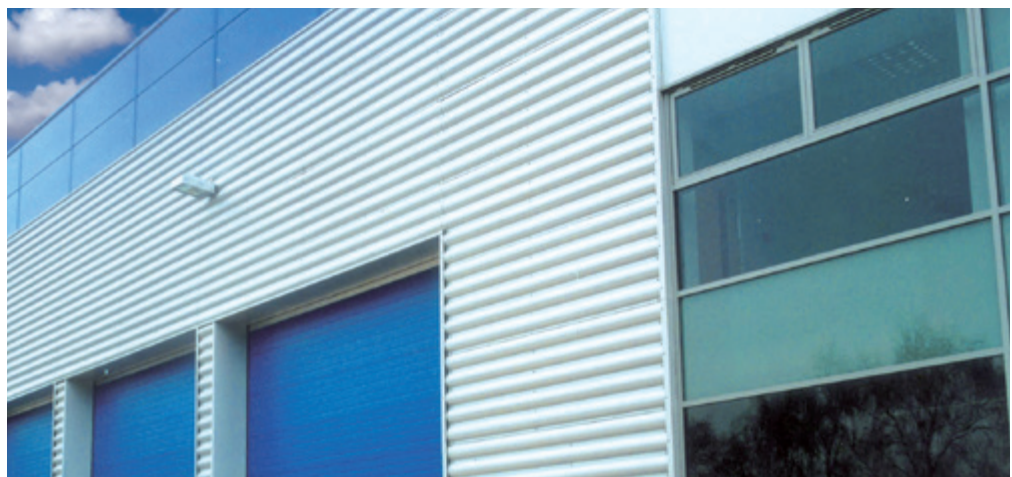
Figure 2.14 Horizontal spanning sheeting
