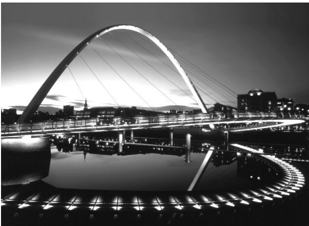
Gateshead Millennium Bridge
