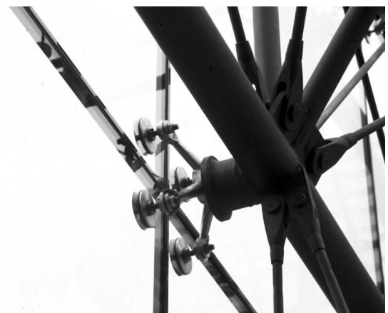
Spider fixing detail
