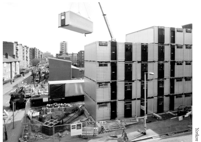
Murray Grove under construction
