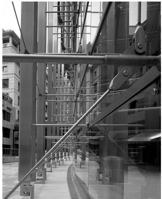
Glazed entrance hall, NatWest Tower, London
