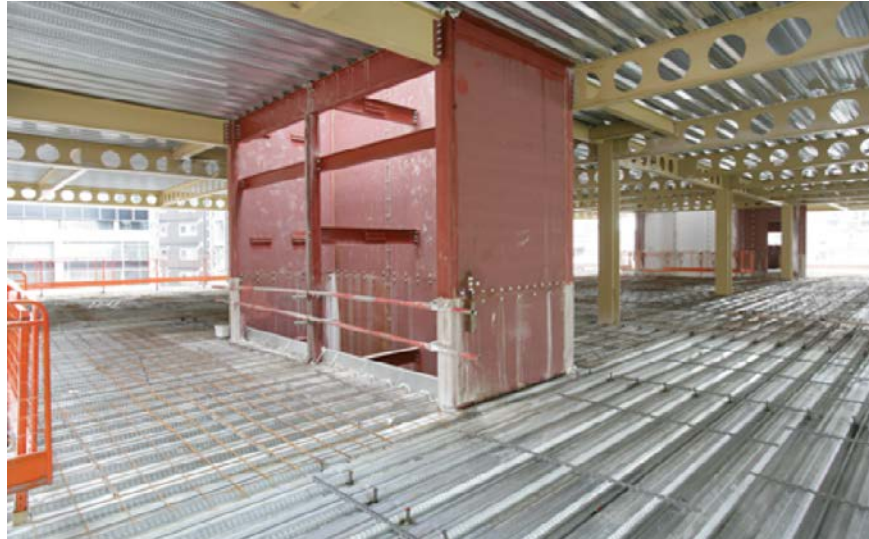
Figure 2.11 – Completed core and floor prior to concreting
