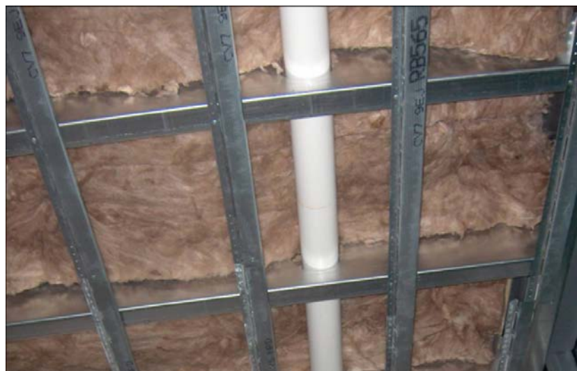
Figure 4.12 – Services passing through light gauge floor steelwork.
