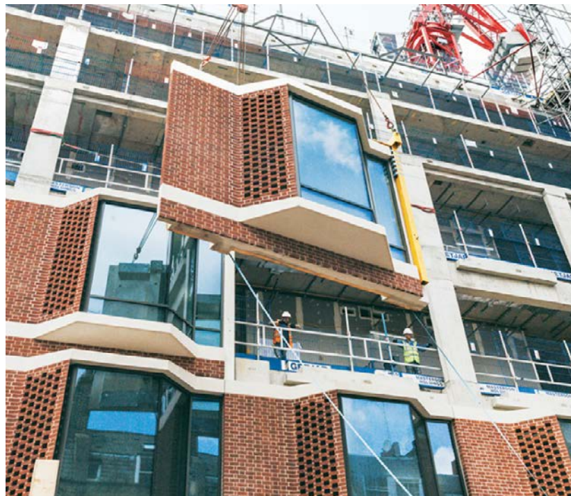
Figure 4.14 – Prefabricated façade panel, University College London Hospital
